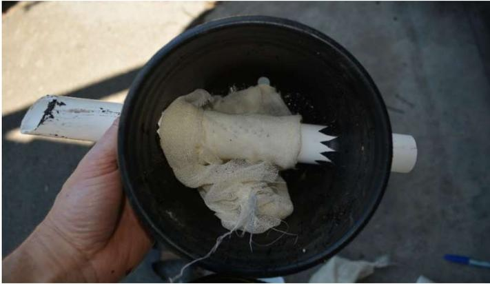
To keep out dirt, wrap a very thin cloth (such as a cheesecloth) over the holes in the pipe.
